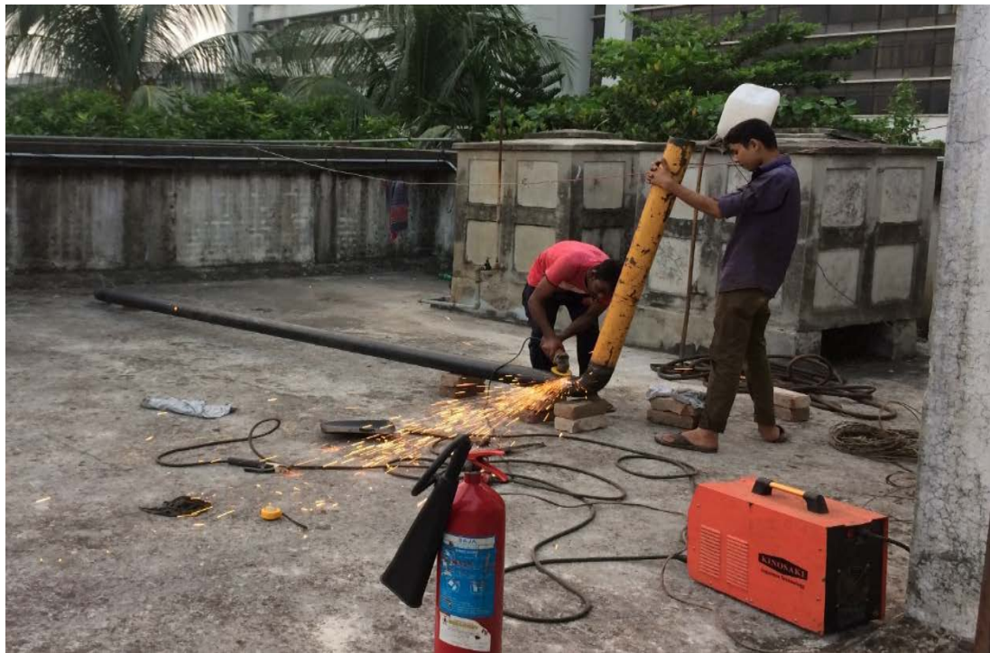
Figure 4.2: Twenty Feet Iron Pipe [Mild Steel] Preparation.
